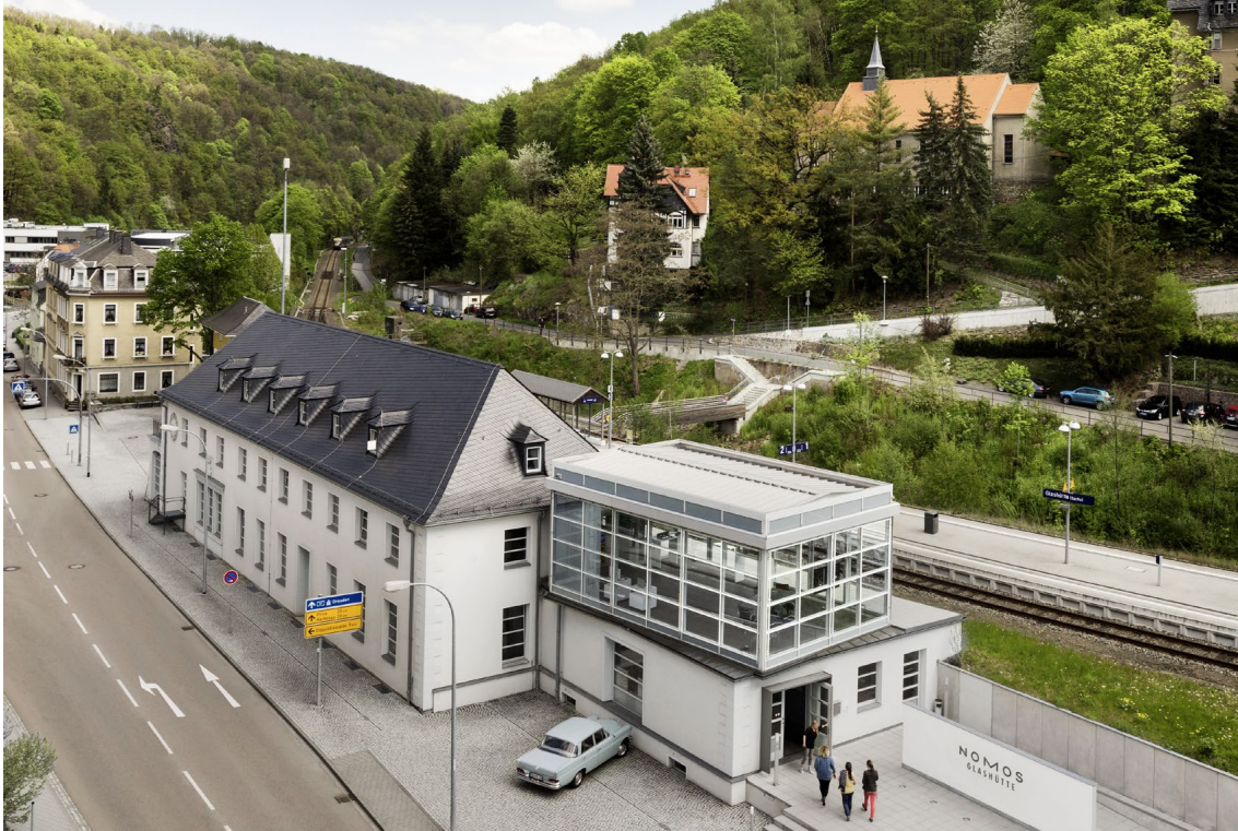
NOMOS headquarters in the former train station of Glashütte
